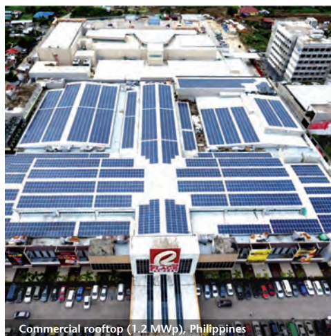
Commercial rooftop (1.2 MWp), Philippines
