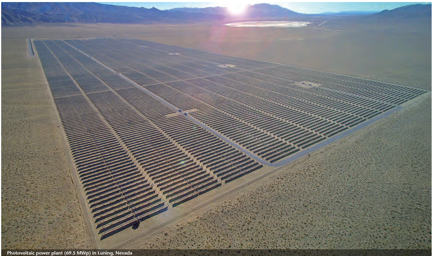
Photovoltaic power plant (69.5 MWp) in Luning, Nevada
